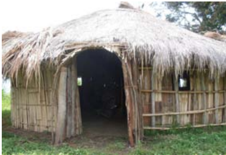
Image 2: A shrine under construction in Kakuka parish, Bundibugyo, 2009
